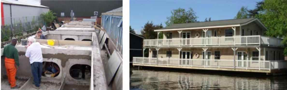
**Figure 28: Construction of a Concrete Pontoon and floating ferro-cement structure along the river Thames. Source AquaBase.**
