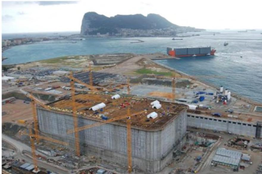
**Figure 133: Construction of a concrete box for the LNG terminal “Adriatic” in Algeciras.
