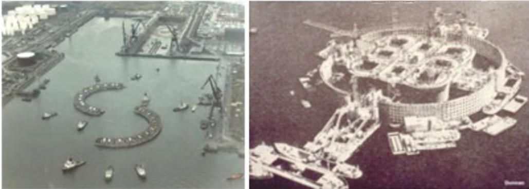
Figure 138: Breakwaters constructed separately and under construction around the structure.
