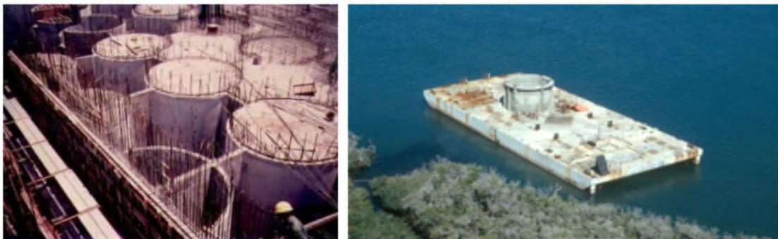
Figure 149: Barge Rofomex I: under construction, Honeycomb system in sight, and afloat (76)
